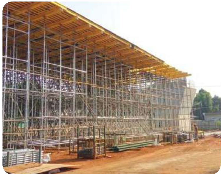
Becakayu Toll Road Project Bekasi, Indonesia.
