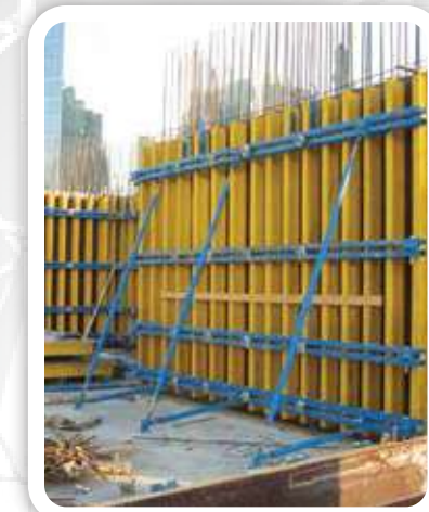
Wall & Column Formwork
